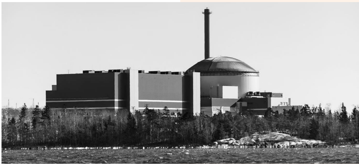
Olkiluoto 3 i Finland.
